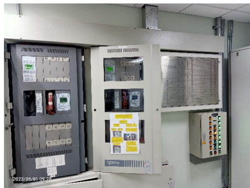
fire alarm control Panel
